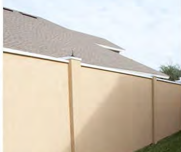
Stucco Concrete Wall
