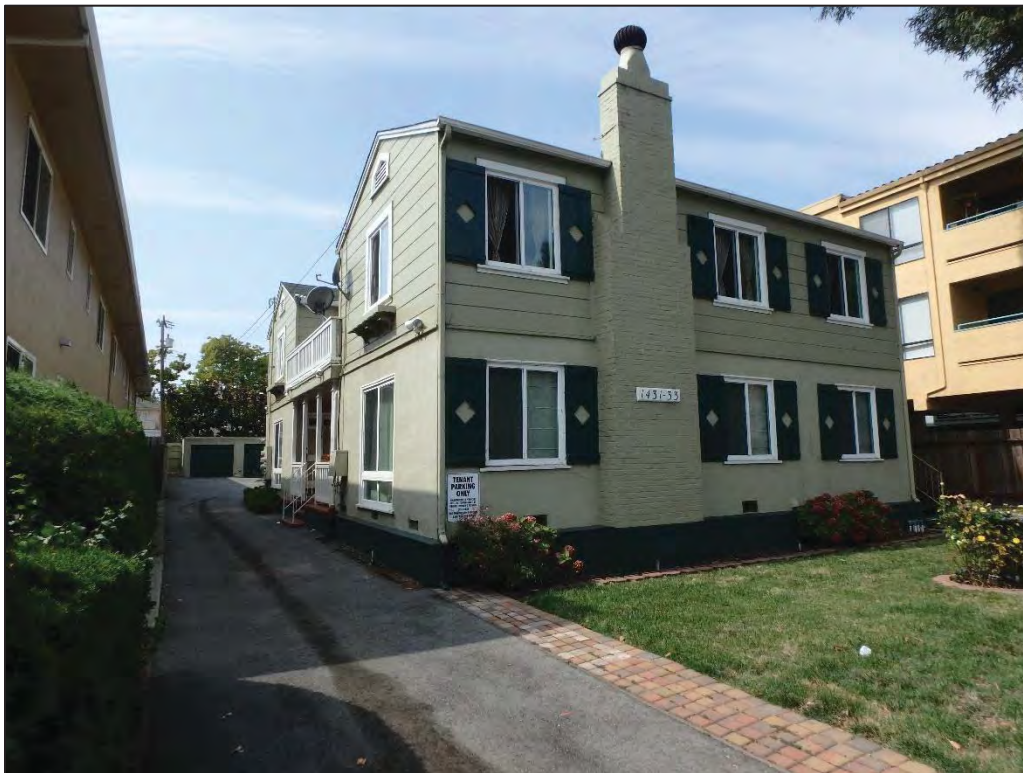
Figure 1. Overview of Northeast Elevation (View To West) IMG #: P9060008
