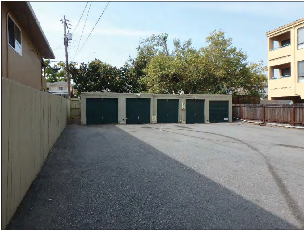
Figure 6. Garage Located to Rear of Building (View to Southwest) IMG#: P9060012
