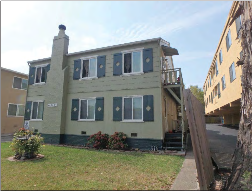
Figure 4. Overview of the Northeast and Northwest Elevations (View to South) IMG #: P9060006
