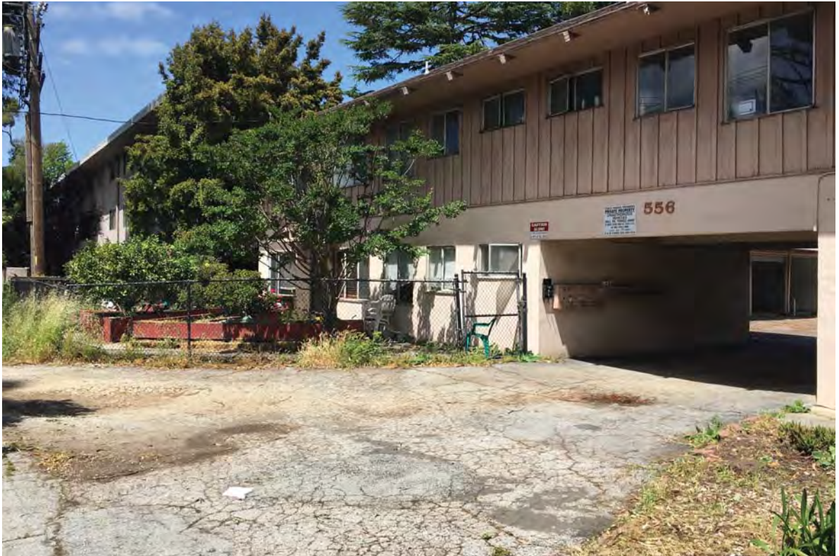
PHOTO 1: View of the project site looking northeast from El Camino Real.
