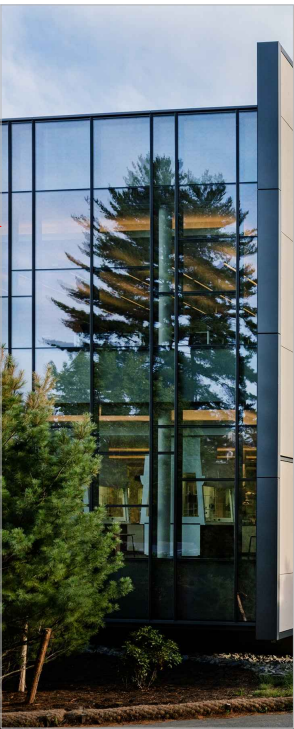
STAIRCASE FACADE: VERTICAL FRAMED GLASS FACADE WITH MULLIONS EMPHASIZE THE BUILDING VERTICALITY AND BREAK THE BUILDING INTO TWO BLOCKS
