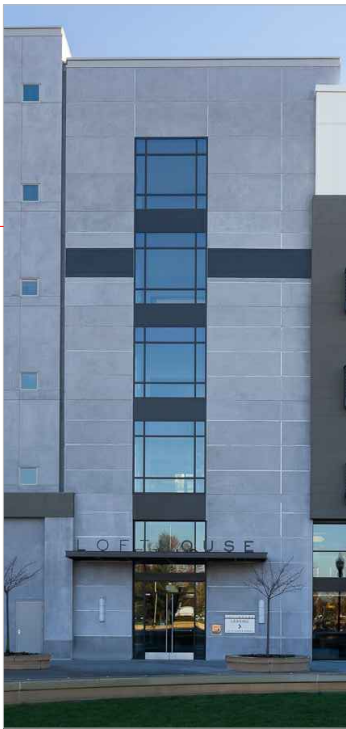
STAIRCASE FACADE: VERTICAL FRAMED GLASS FACADE WITH MULLIONS EMPHASIZE THE BUILDING VERTICALITY AND BREAK THE BUILDING INTO TWO BLOCKS
