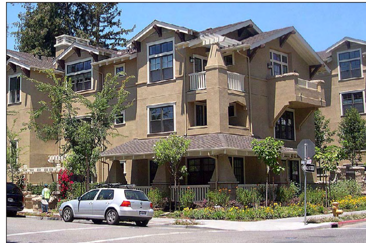
FIGURE 5-27: Buildings should contribute to an appealing neighborhood character and should employ recognizable residential design details such as visible residential entries, porches, bay windows and roof overhangs, and balconies and small outdoor areas.
