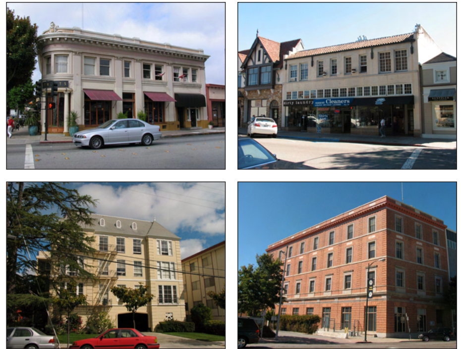
FIGURE 5-44: Downtown's late 19th and early 20th Century buildings contribute historic character and distinctiveness to this desirable pattern and mix of buildings.
