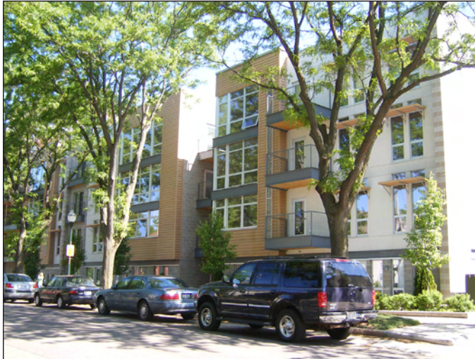
FIGURE 5-30: Articulation, setbacks, and materials should minimize massing, break down the scale of buildings, and provide visual interest.
