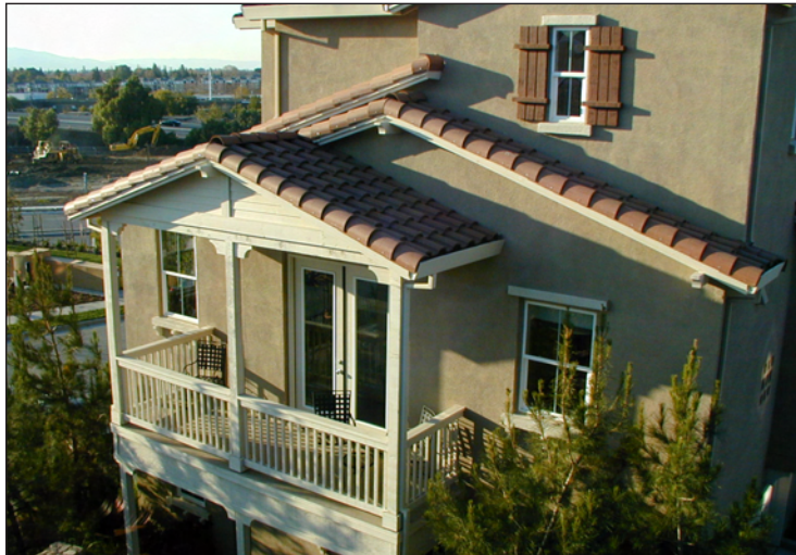
FIGURE 5-34: Windows should be inset generously from the building wall to create shade and shadow detail.
