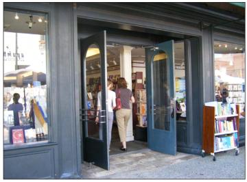
FIGURE 5-3: Commercial entrances should be recessed from the facade, creating a small alcove.
