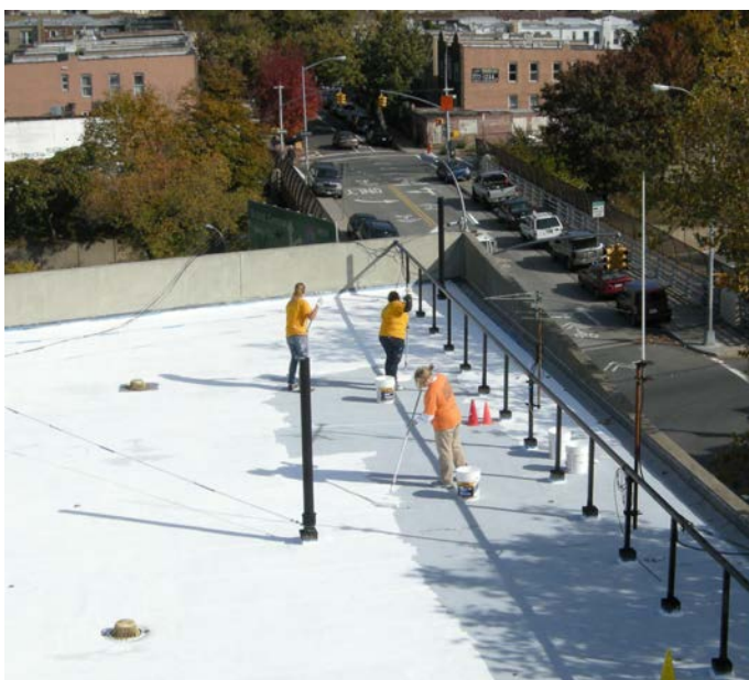
Example: Cool Roof Installation
