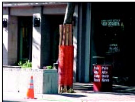
IMAGE 2.15-4 Trunk Wrap Protection
