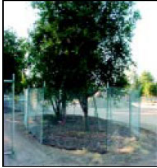
IMAGE 2.15-1 Tree Protection Fence at the Dripline
