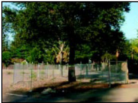
IMAGE 2.15-2 Tree Protection Fence at the Dripline
