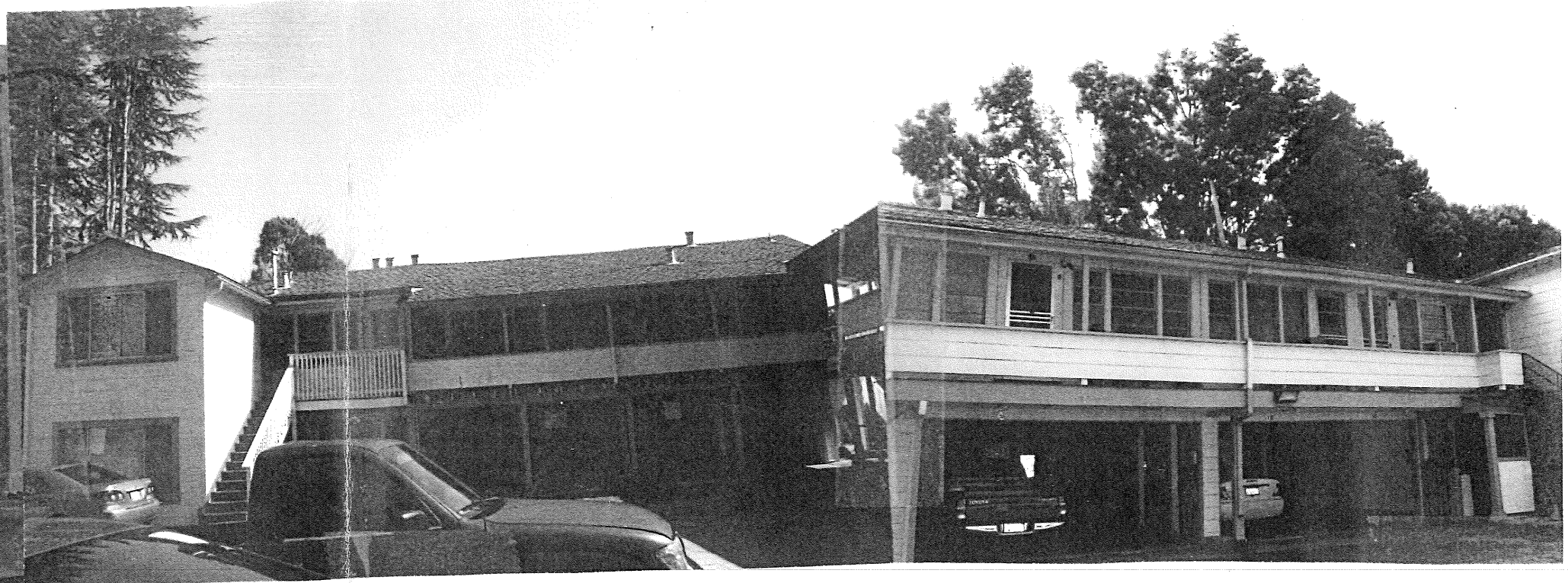
1509 El Camino (Pano view) at the rear of lot
