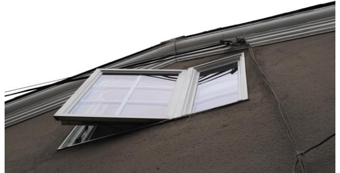
Figure 10. Non-original vinyl-sash window with simulated divided lites at the gable peak on the north façade.
