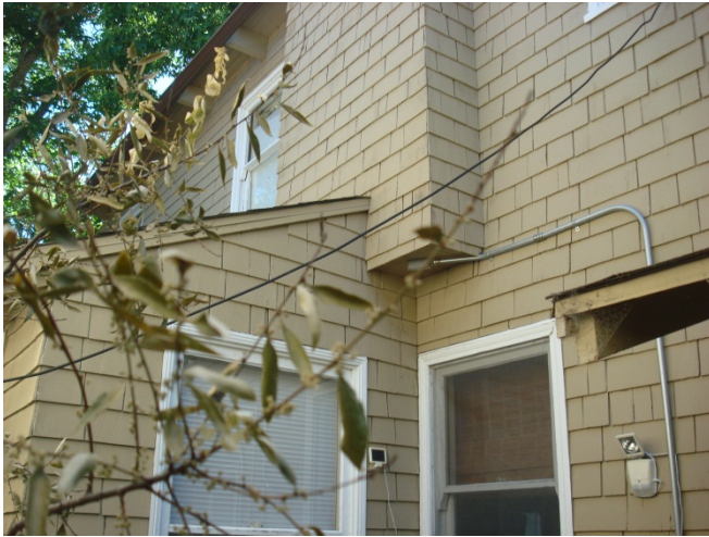
Figure 3: North (rear) facade, partial view. (Page & Turnbull, May 2013)
