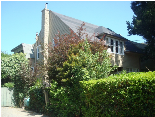
Figure 1: 1128 Douglas Avenue, west facade. (Page & Turnbull, May 2013)
