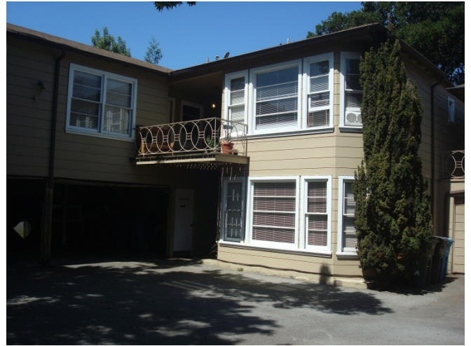
Figure 4: Apartment behind subject property. (Page & Turnbull, May 2013)
