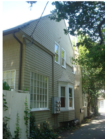
Figure 2: 1128 Douglas Avenue, east facade. (Page & Turnbull, May 2013)
