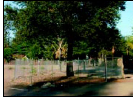
IMAGE 2.15-2 Tree Protection Fence at the Dripline
