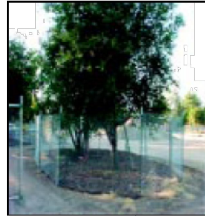
IMAGE 2.15-1 Tree Protection Fence at the Dripline
