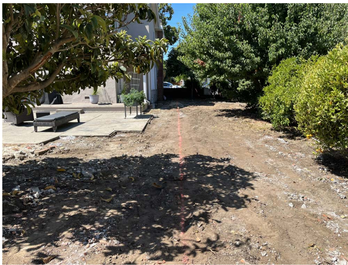
3 Planting Area / Concrete Demo
