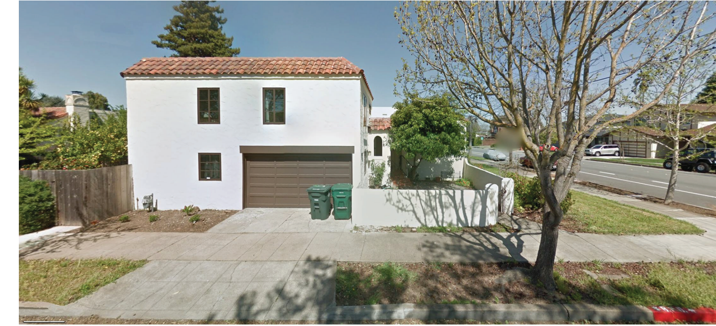
SUBJECT PROPERTY 520 HOWARD AVENUE
