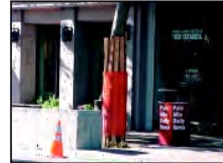
IMAGE 2.15-4 Trunk Wrap Protection
