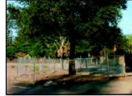
IMAGE 2.15-2 Tree Protection Fence of the Dripline
