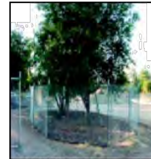
IMAGE 2.15-1 Tree Protection Fence of the Dripline
