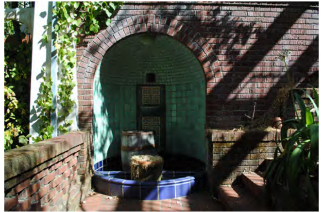
Figure 25. Inset arched fountain with decorative tiles at the southwest corner of the rear façade.
