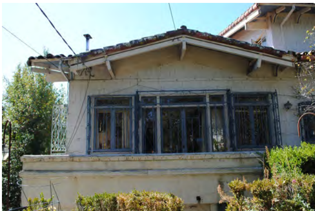
Figure 3. Easternmost volume of the primary façade, facing south.
