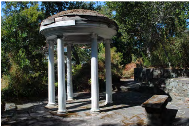
Figure 44. Gazebo structure and concrete bench located in a hardscaped area of the site.
