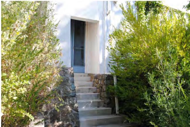
Figure 26. Exterior access door to the upper basement level on the rear façade.
