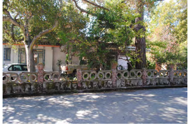
Figure 37. Concrete fence along Hillside Circle featuring texture loops and tree trunk motifs.
