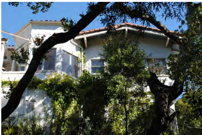
Figure 22. Projecting front-gabled bay at the east end of the rear façade, adjacent the southeast tower.
