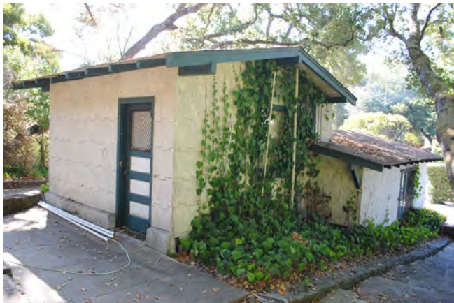
Figure 34. Two gabled masses comprise the detached garage fronting Easton Drive, looking southeast.
