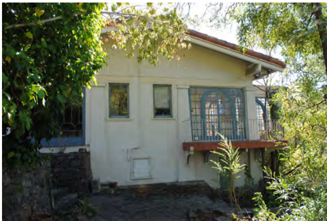
Figure 12. Partial view of the west façade, looking east.
