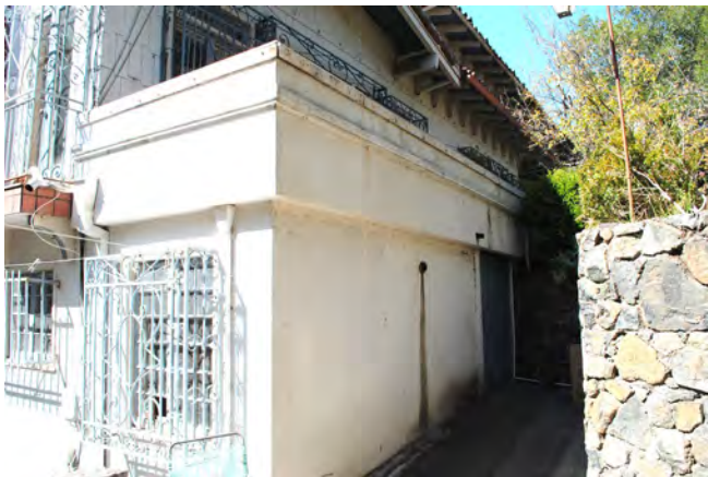
Figure 5. Exposed basement level behind a stone retaining wall at the northeast corner of the residence, looking southwest.
