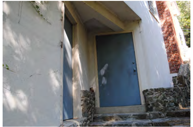
Figure 29. Recessed doors at lower basement level.
