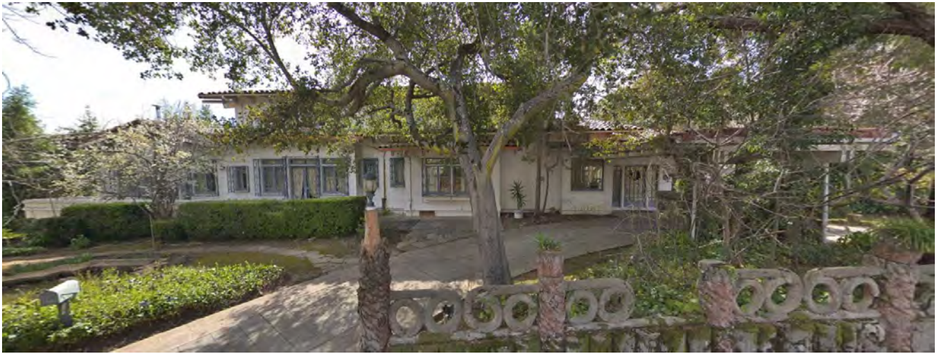
Figure 2: Primary (north) façade of 1385 Hillside Circle, looking south (February 2018). Source: Google Street View, 2018.
