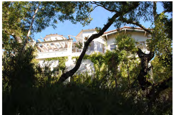
Figure 15. Partial view of east end of west façade, looking up and north.
