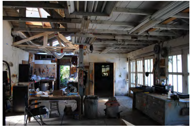
Figure 33. Interior view of garage fronting Hillside Circle, including non-original skylights.
