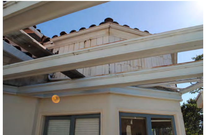
Figure 21. One-story southeast tower has stucco and wood shingle cladding, looking east.
