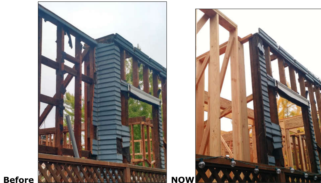
Left Rear - old wall intersects 4-6" LOWER than cantilever top plate
