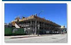
The project consists of eighty residential units in a new 5-story wood framed structure over 3-story concrete podium and associated site improvements. Construction is about 15% complete.
