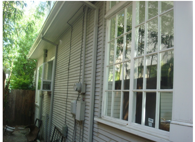
Figure 2: 1132 Douglas Avenue, west façade. (Page & Turnbull, May 2013.)
