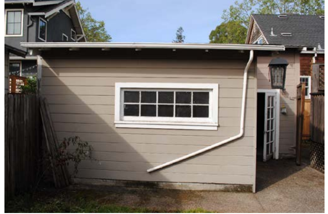
Figure 15. East façade of the detached garage, looking west.
