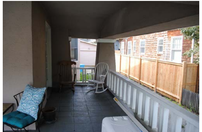
Figure 5. Entry porch, which wraps around to the west façade, looking south.
