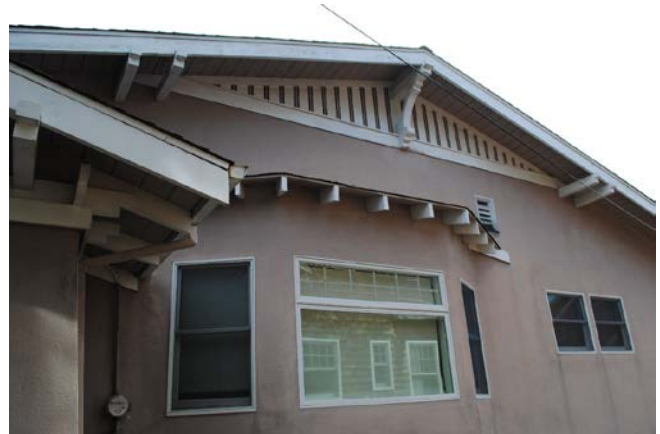
Figure 9. Decorative detailing, wood knee braces, and exposed purlin tails with elaborated ends under the gable of the west façade.
