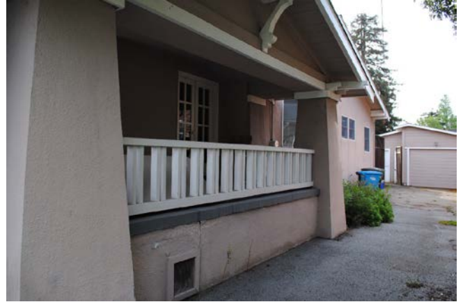
Figure 7. Partial view of the porch on the west façade and the driveway leading to the detached rear garage, looking south.
