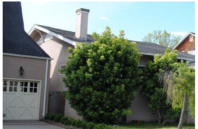
Figure 13. Partial view of the north end of the east façade, looking southwest.
