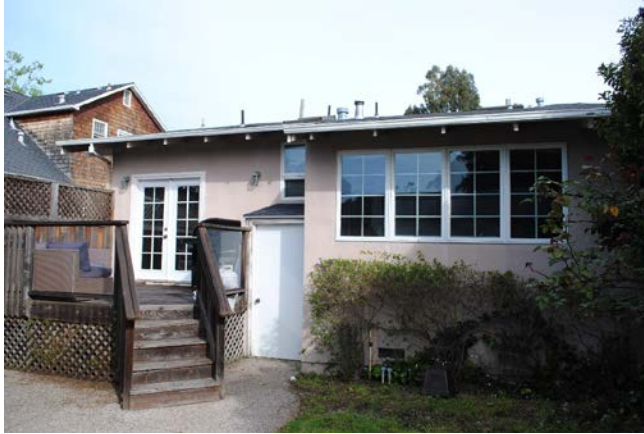
Figure 10. Rear (south) façade, looking north.
