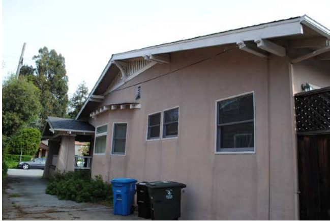
Figure 6. Partial view of the west façade, looking northeast.
