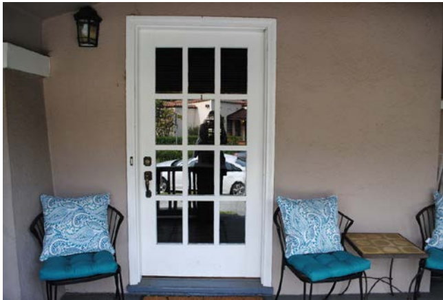
Figure 4. Primary entry door, located on the primary (north) façade, looking south.
