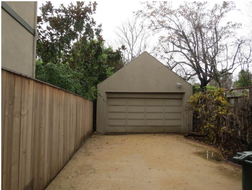
Figure 10. Garage, east (primary) façade, with fenced rear yard at right. Page & Turnbull, December 2014.
