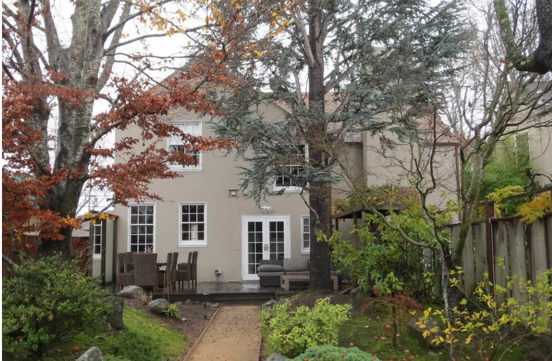
Figure 6. West (rear) façade, showing one of the two rear entries and the chimney at right (partially obscured by trees). Page & Turnbull, December 2014.
