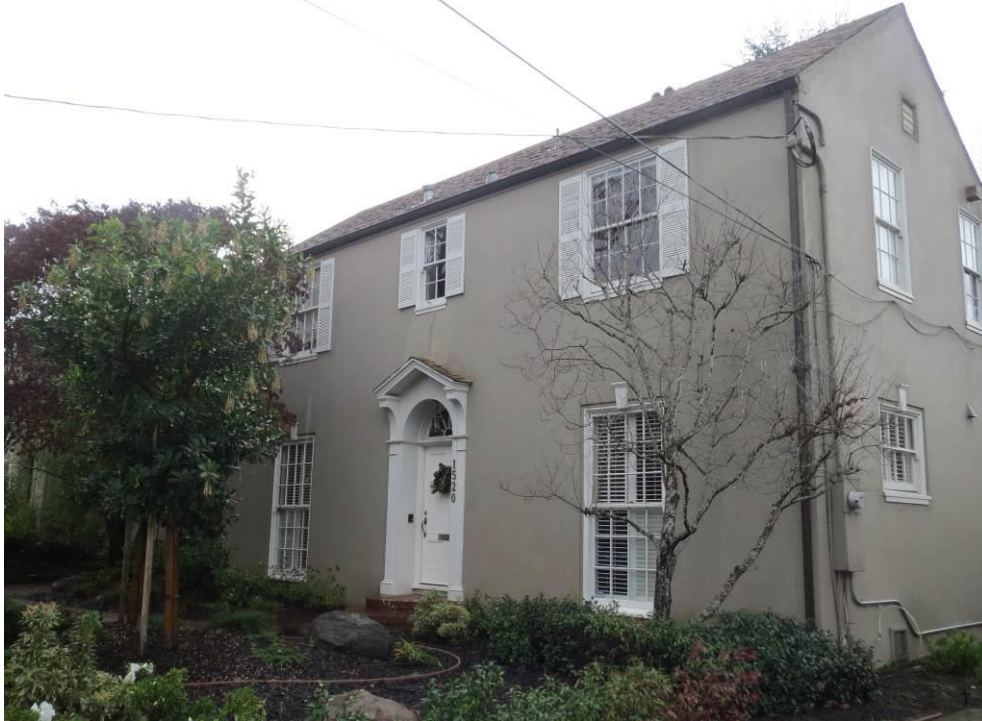
Figure 1. Primary (east) façade, looking southwest on Cypress Ave. Page & Turnbull, December 2014.
