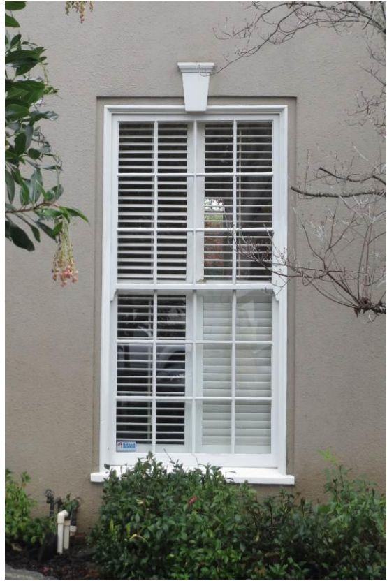
Figure 4. Detail of window on east facade. Page & Turnbull, December 2014.
