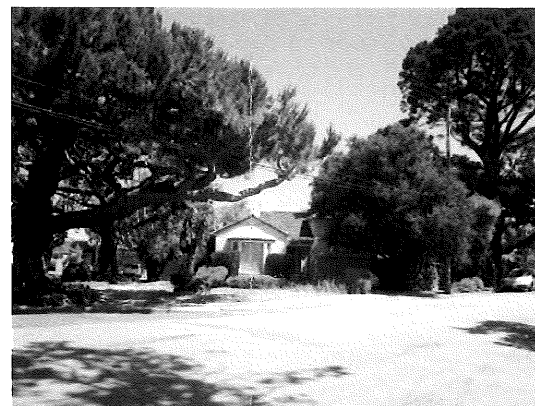
524 Oak Grove Ave. (subject property)
