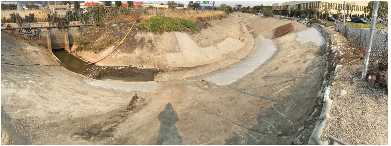
Post construction - El Portal Channel – concrete repairs completed
