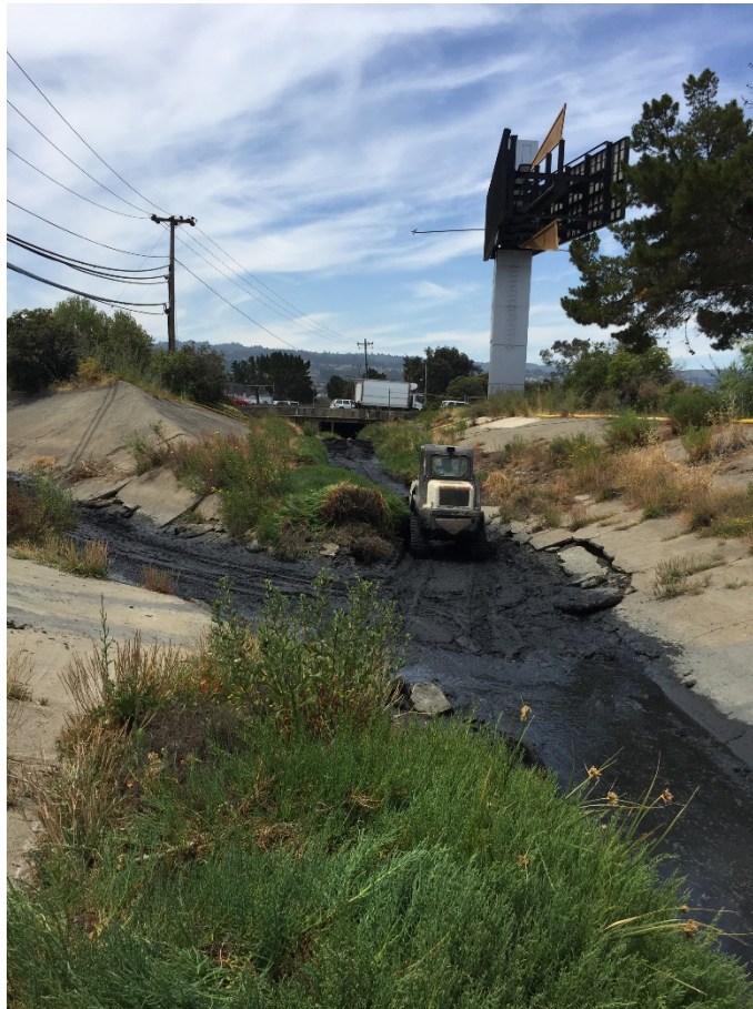
During construction - El Portal Channel merge with Trousdale Channel at HWY 101 – removal of sludge
