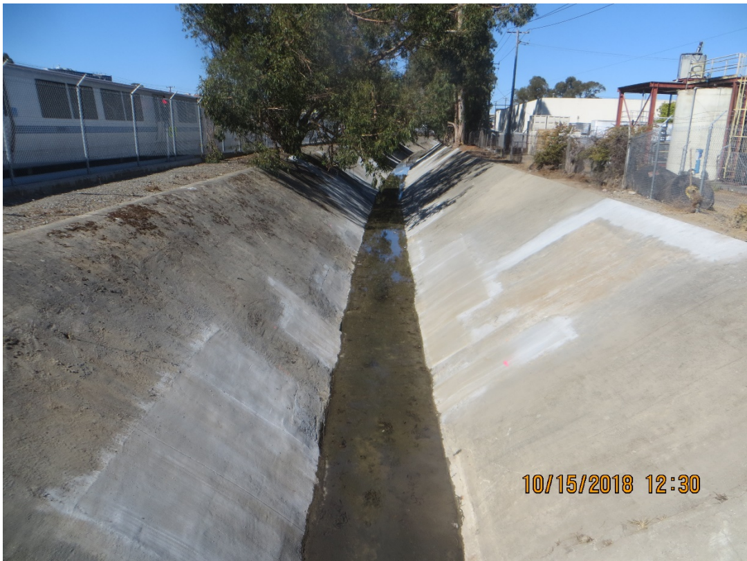
Post-construction - Trousdale Channel – removal of trees and repaired concrete areas
