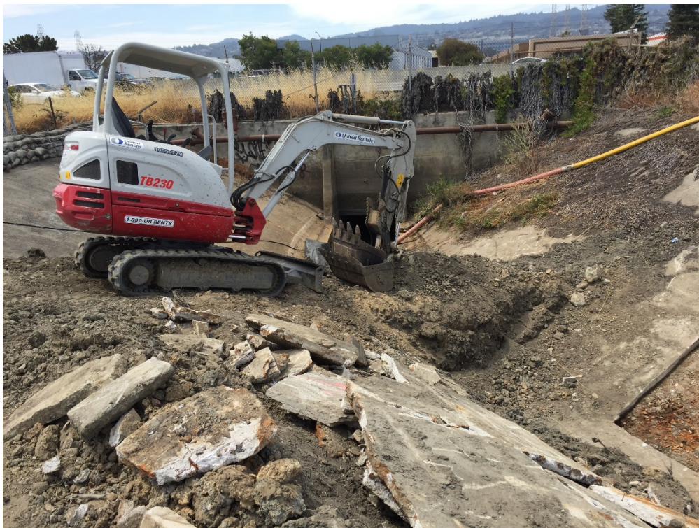
Construction – removal of deteriorated concrete at El Portal Channel
