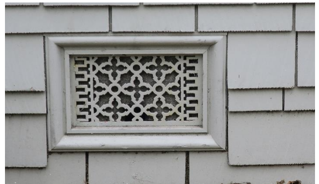
Figure 4: Metal vent grille beneath south window.
