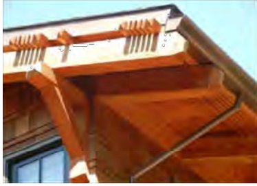
Building with copper flashing, gutter and drainpipe.
