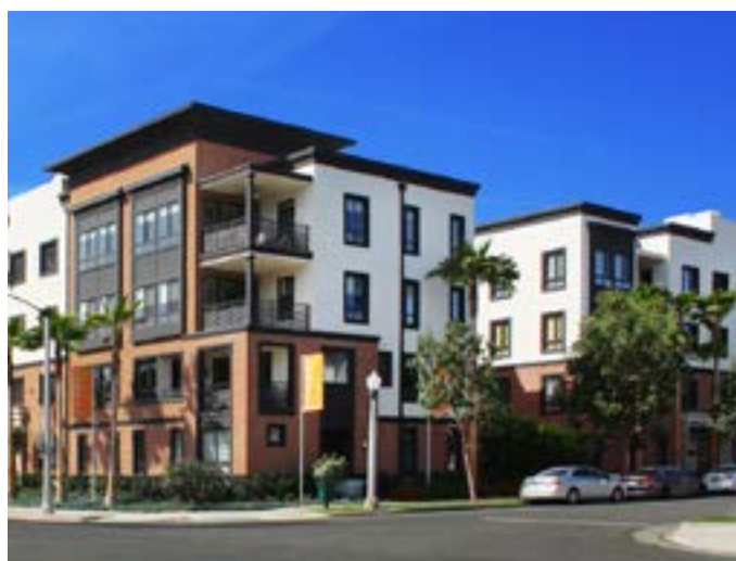
Example: Stacked flat building. Single-level floorplates are vertically stacked and accessed from a central lobby and parking area.
