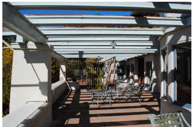
Figure 23. Rear porch covered by a wood trellis, supported by battered columns. Stairs down to the rear garden are located toward the west end of the porch.
