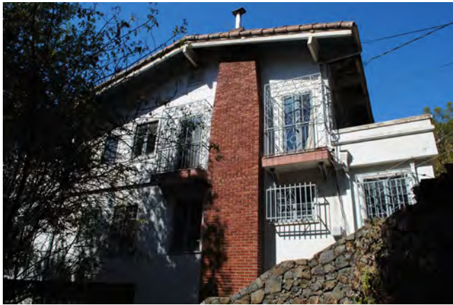
Figure 28. Partial view of east façade, looking west.
