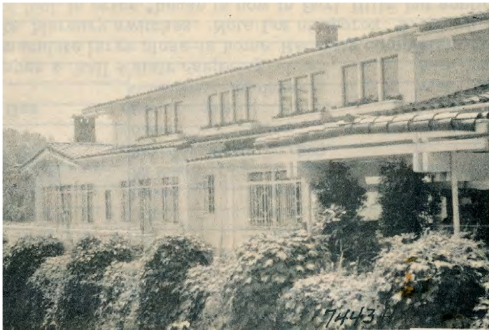
Figure 58. 1385 Hillside Circle, looking southeast toward primary façade (June 1963). Source: Burlingame Historical Society.
