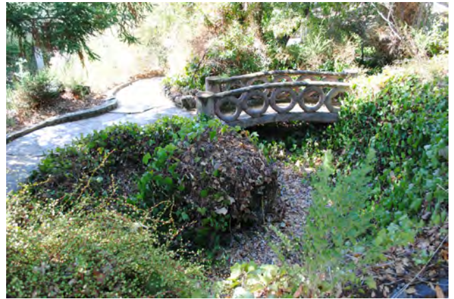
Figure 43. Concrete bridge over what appears to be an overgrown, former water feature.
