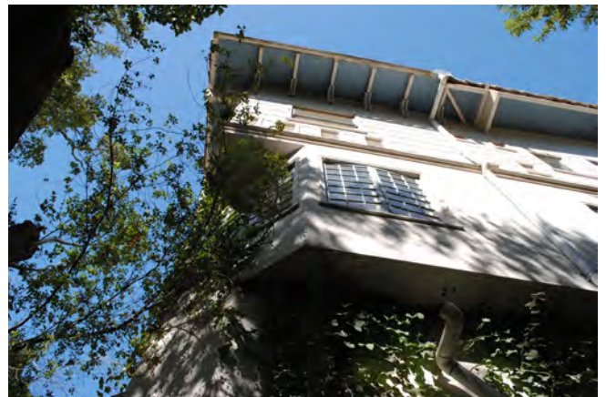
Figure 27. Southeast corner with chamfered sides at the two basement levels.
