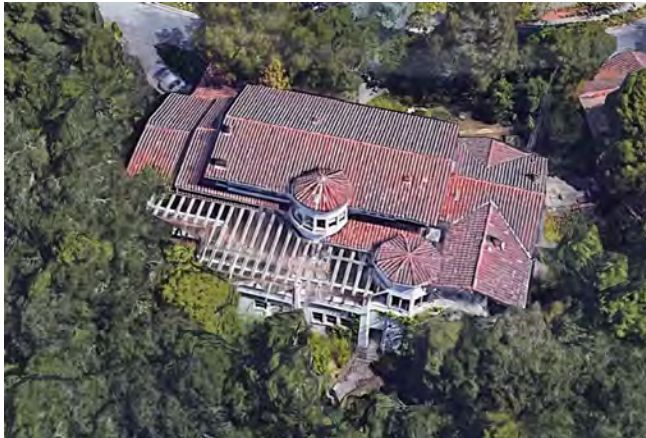
Figure 14. Bird's-eye view of the rear (south) façade of 1385 Hillside Circle. Source: Google Maps, 2018.
