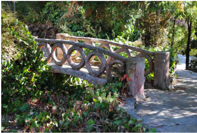
Figure 42. One of two concrete bridges with decorative railings with posts textured to resemble tree trunks.
