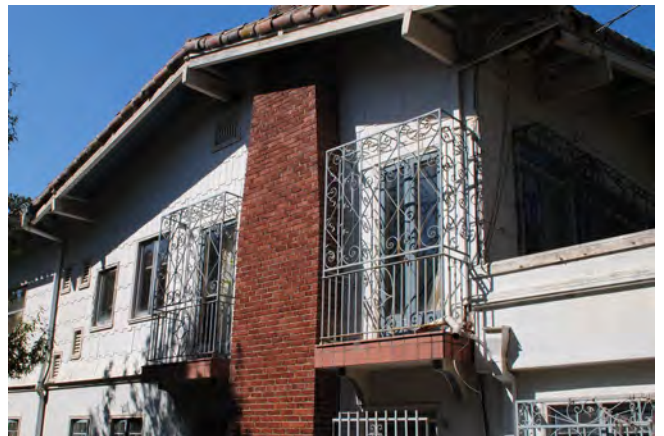
Figure 31. Enclosed balconettes on the east façade, looking west.
