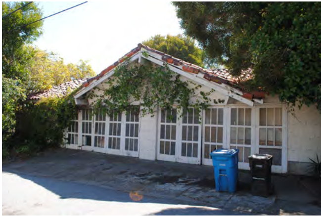
Figure 32. Detached garage fronting Hillside Circle, looking south.
