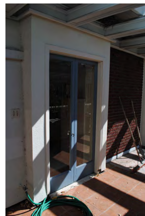
Figure 17. Typical double-doors and exterior brick chimney.
