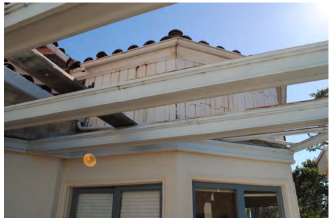
Figure 21. One-story southeast tower has stucco and wood shingle cladding, looking east.
