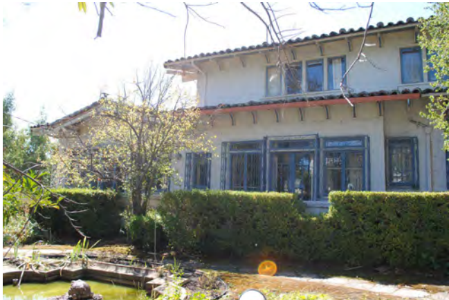
Figure 6. Partial view of central, two-story volume at primary façade, looking southeast.
