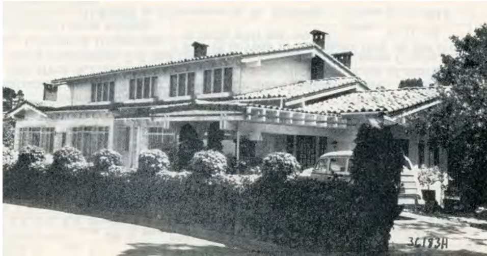
Figure 57. 1385 Hillside Circle, looking southeast toward primary (north) and west facades (June 1963). Source: Burlingame Historical Society.
