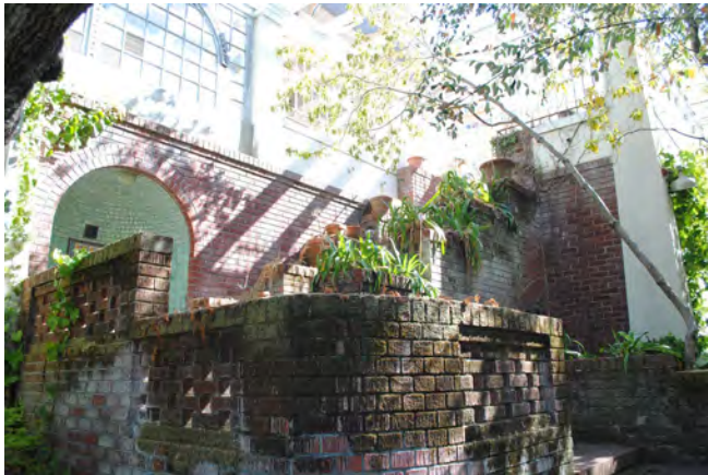
Figure 24. Brick steps leading down from rear porch down to the rear gardens.
