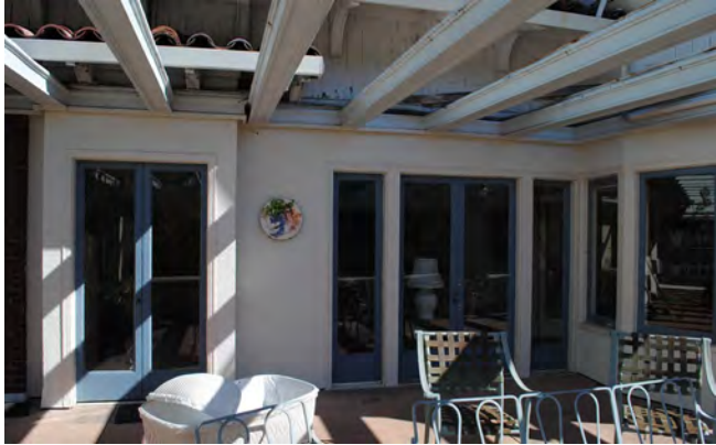
Figure 18. Typical double-doors with sidelites adjacent tower.
