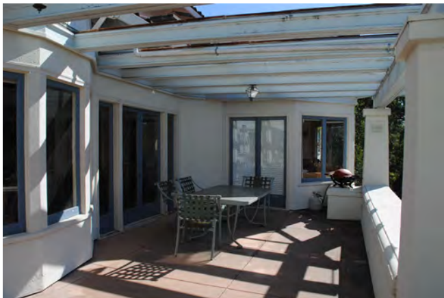
Figure 20. One-story tower at east end of the rear porch, looking east.
