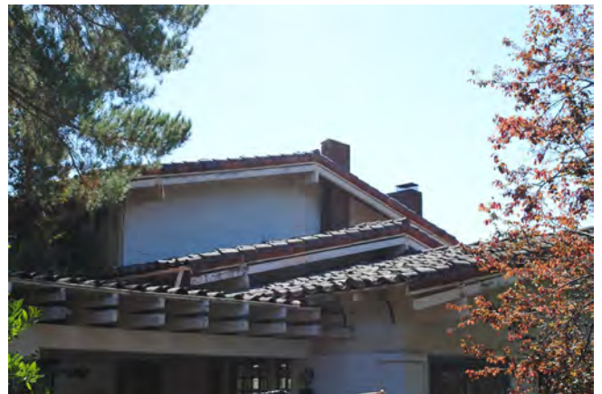
Figure 13. Detail view of staggered roof forms above the west façade, looking southeast.
