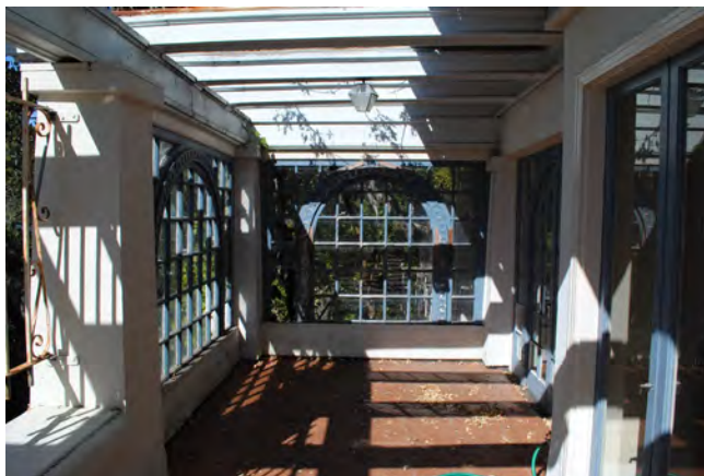
Figure 16. West end of rear façade, looking west.
