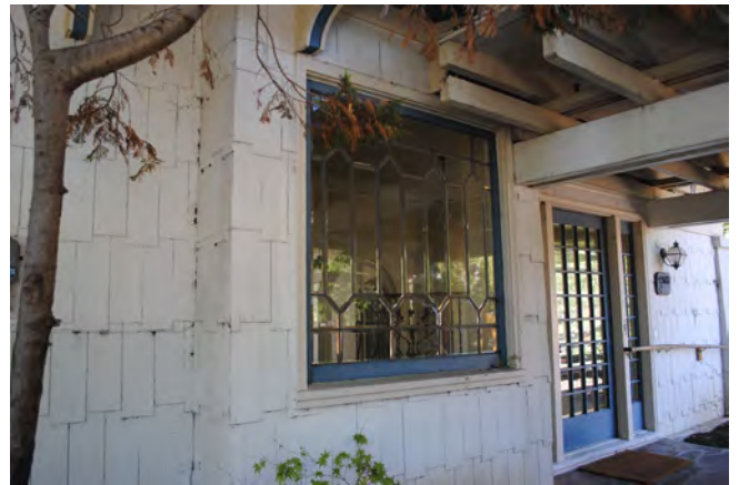
Figure 9. Fixed, leaded glass window adjacent the primary entrance, looking southwest.
