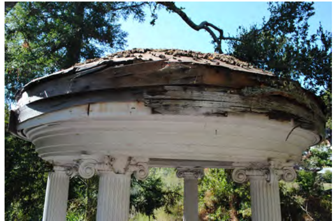
Figure 45. Concrete Classical columns support the wood domed roof of the gazebo.
