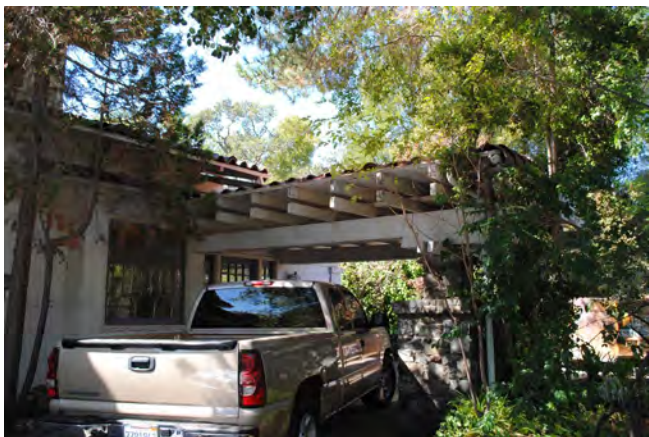
Figure 10. Port-cochere at main entrance on the westernmost volume on the primary façade, looking southwest.
