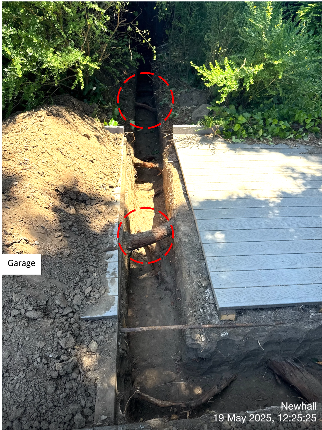
Photo 3. Garage side of "L" shaped excavation. Two roots (circles) in the top 12" of the soil profile must be severed to allow garage construction. Anticipated impact is minimal. Root at the bottom right is from Tree #2 (proposed for removal).
