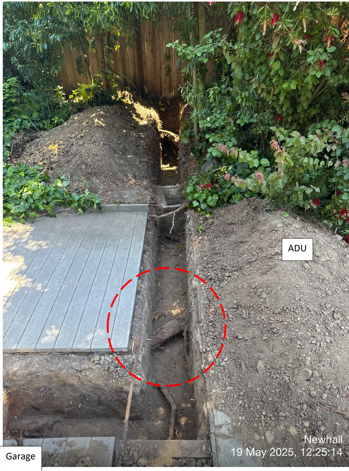
Photo 2. ADU side of “L” shaped excavation. One large root (red circle) was discovered and determined to belong to Tree #2, based on its orientation and taper relative to the three redwoods.
