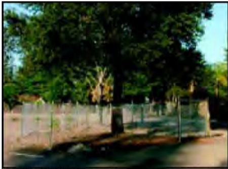
IMAGE 2.15-2 Tree Protection Fence at the Dripline
