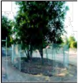
IMAGE 2.15-1 Tree Protection Fence at the Dripline
