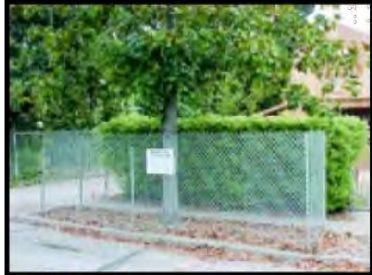
IMAGE 2.15-3 Tree Protection within a Planter Strip
