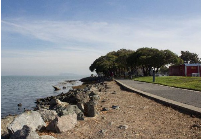
PROTECT – ENGINEERED Coastal armoring, seawalls and levees, Burlingame
