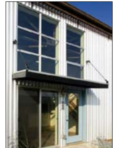
FIGURE 5-11: Design features such as corrugated metal roofs and sidings, simple multi-paned metal rimmed windows, and recycled "green" building materials can maintain the existing varied character of the Myrtle Road Mixed Use Area.
