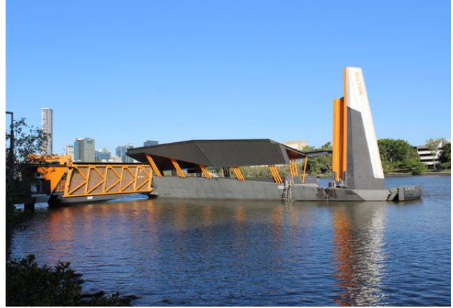
ADAPTATION Flood resilient ferry wharf, Brisbane Australia
