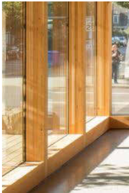
8) WINDOW MULLIONS - 5TH FLOOR, INTERIOR WOOD MULLIONS
