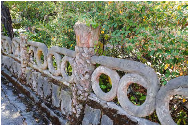
Figure 38. Concrete post, also textured to resemble a tree trunk, is attached to the top of the post.
