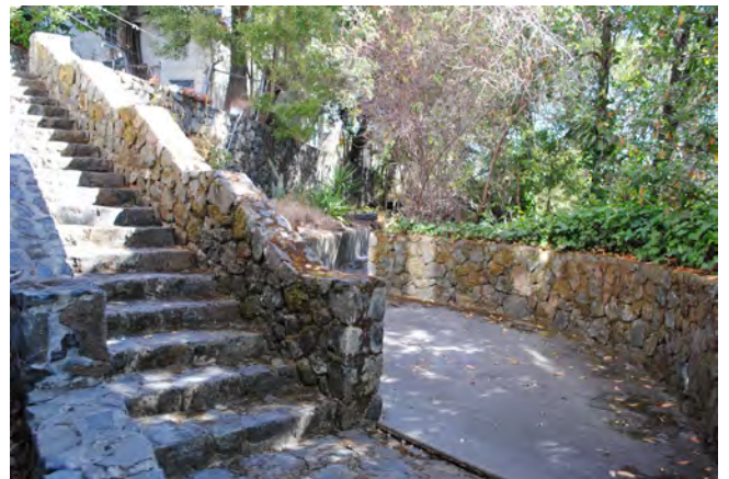
Figure 41. Concrete path located east of the stairs running along the east façade of the main residence.
