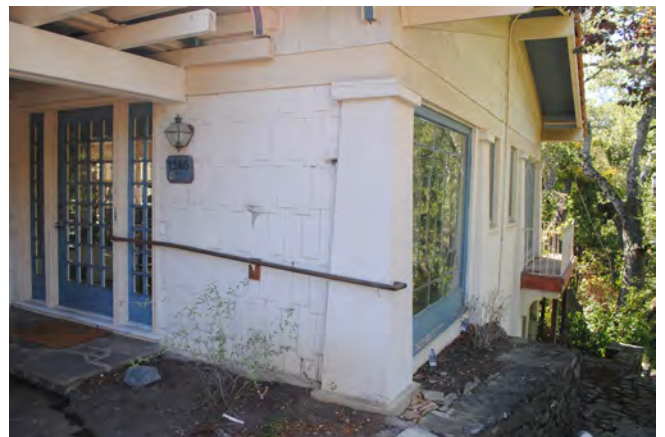
Figure 11. Primary entrance and engaged battered column at the northwest corner of the primary façade, looking south.
