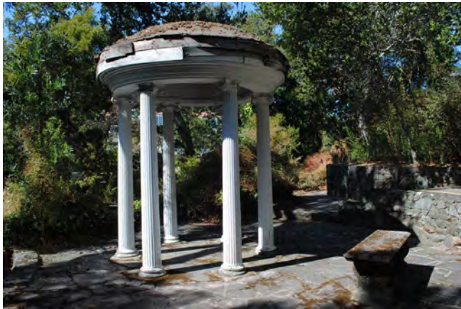
Figure 44. Gazebo structure and concrete bench located in a landscaped area of the site.
