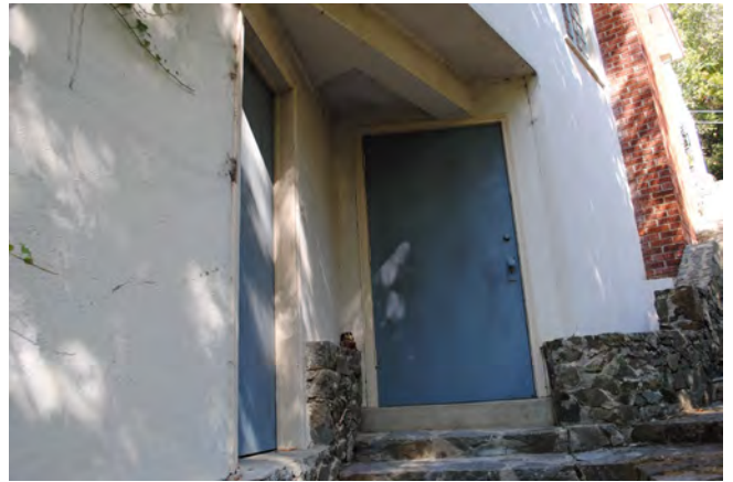
Figure 29. Recessed doors at lower basement level.
