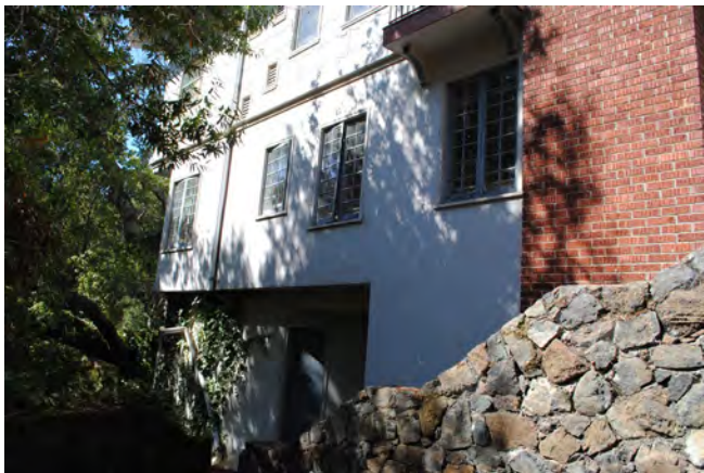
Figure 30. Multi-lite casement and double-casement windows at upper basement level, looking southwest.
