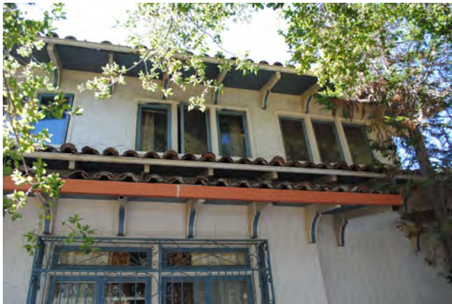
Figure 8. Two banks of three typical casement windows at the second story of the central volume, looking south.
