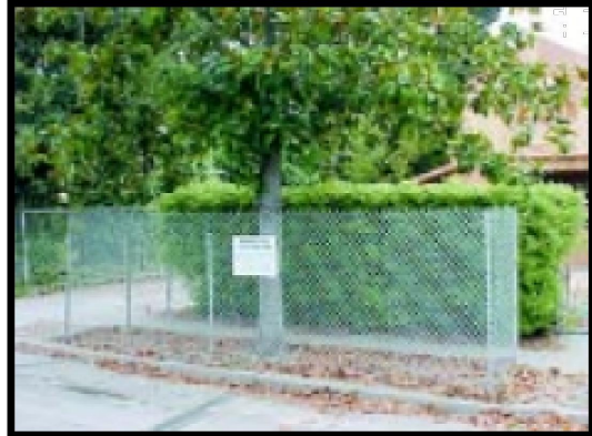
IMAGE 2.15-3 Tree Protection within a Planter Strip
