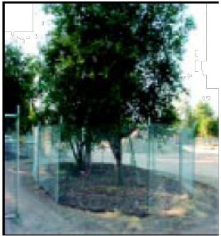
IMAGE 2.15-1 Tree Protection Fence at the Dripline
