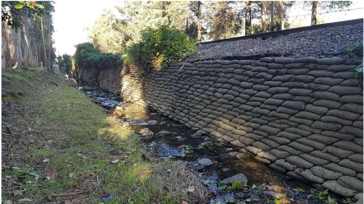
Photo 1. Burlingame Creek, looking downstream to the west. Channel is approximately 6 feet wide and not subject to tidal action. The channel will be maintained by pushing debris and leaf litter from the eucalyptus trees lining the banks with a bobcat into an excavator bucket and haul trucks.
