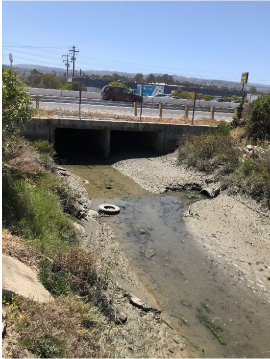
Mills Creek (Reach 4) immediately east of Hwy 101 North.
