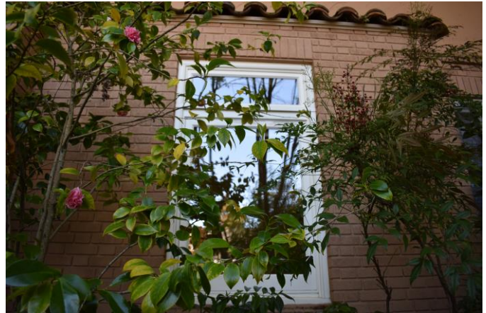
Figure 6. Projecting bay with fixed vinyl window and transom, looking south.
