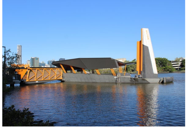
ADAPTATION Flood resilient ferry wharf, Brisbane Australia
