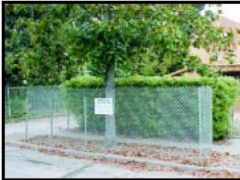
IMAGE 2.15-3 Tree Protection within a Planter Strip
