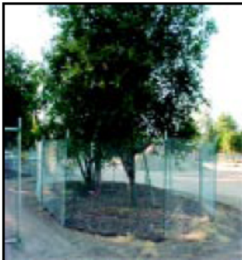
IMAGE 2.15-1 Tree Protection Fence at the Dripline
