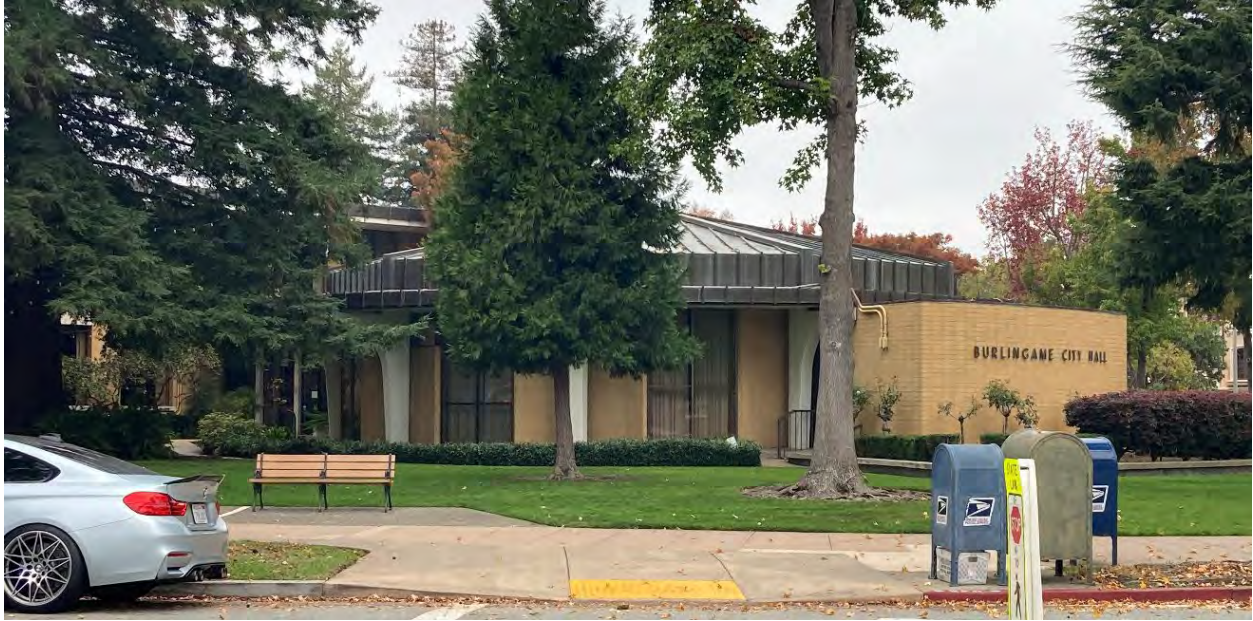
Note: The caucus room occupies the small room visible at the far right. Source: ESA, 2025
