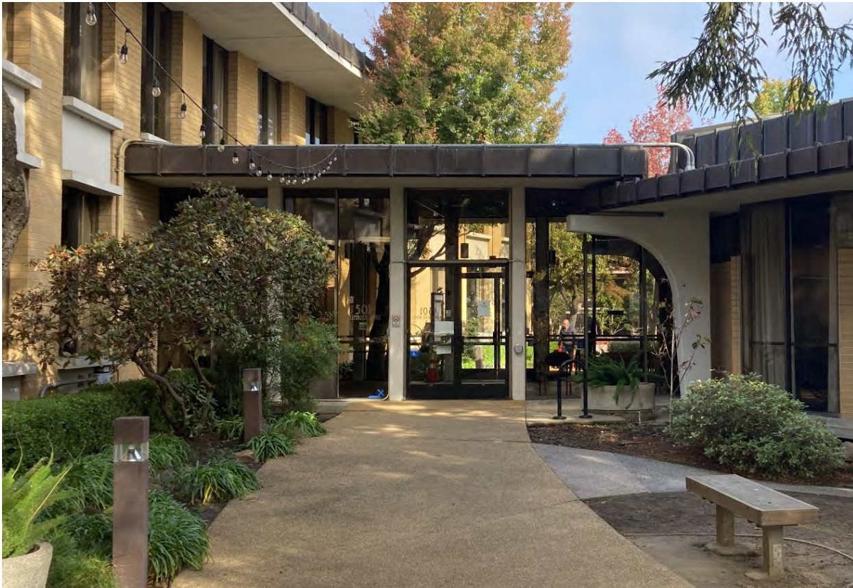
South façade of the lobby, view facing north. The administrative offices are visible on the left, and the council chamber is visible on the right. Source: ESA, 2025.
