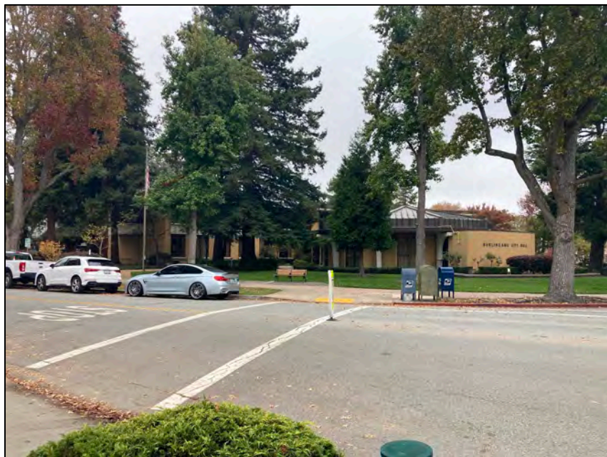
P5b. Description of Photo: Overview of Burlingame City Hall, facing north from Bellevue Avenue. Source: ESA, 2025.
