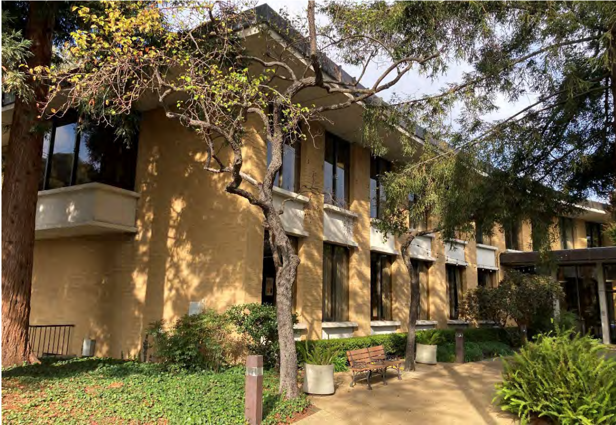
Primary (east) façade of the administrative offices, south end, view facing northwest. The lobby is partially visible on the right. Source: ESA, 2025.
