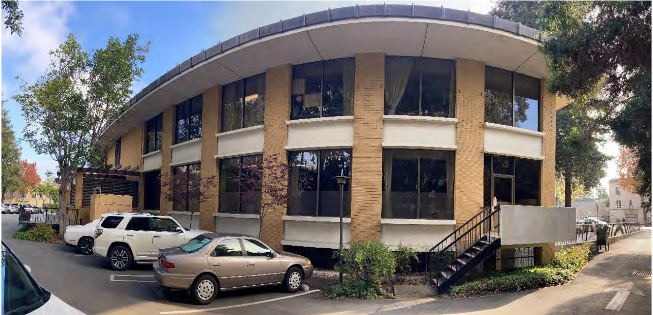
Rear (west) façade of the administrative offices, south end, view facing east. Source: ESA, 2025.
