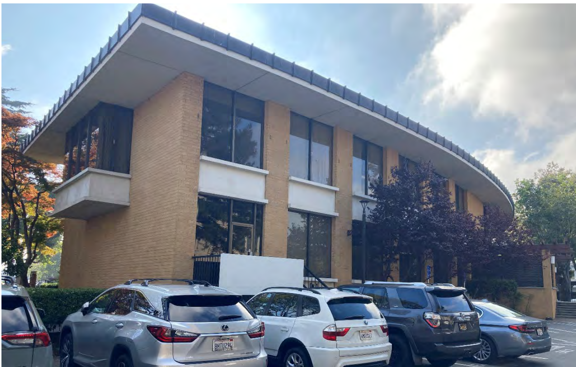
Rear (west) façade of the administrative offices, north end, view facing southeast. Source: ESA, 2025.
